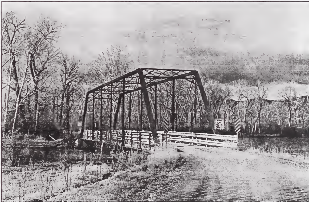
Looking Southwest at East Approach
